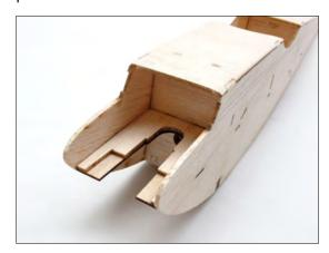
Fit and glue F7 to notches in front of fuselage assembly.
